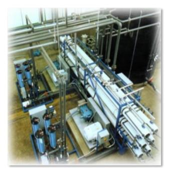
In 1996 the FTS technical team delivered a 150 m3/day leachate treatment facility with primary objectives of high permeate quality and water recovery > 90%
